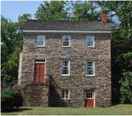
Figure 15: Buckland Tavern is one of several early-19 th -century structures contained within the Buckland Historic District.
