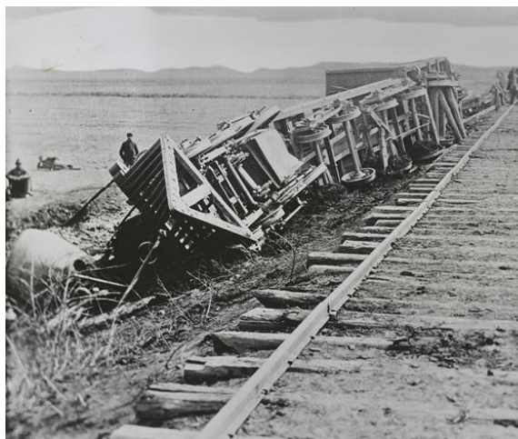
Figure 27: Train derailed by Confederate cavalry during the Manassas Station Operations, August 26, 1862. Andrew J. Russell 58 .
